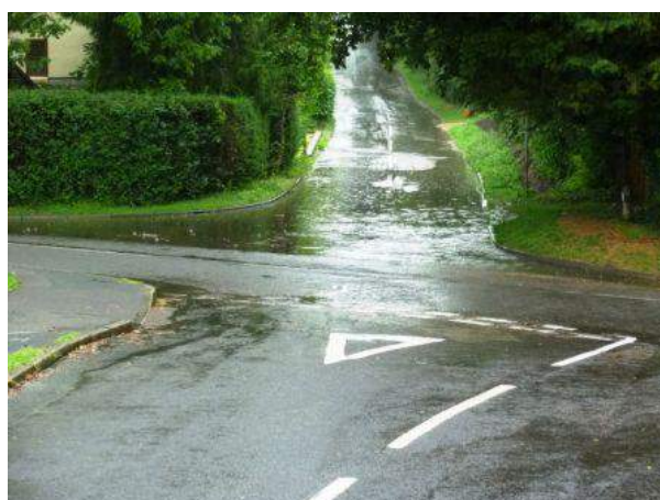
Lymington Bottom at its junction with Brislands Lane highlighted as an area with regular flooding problems.
