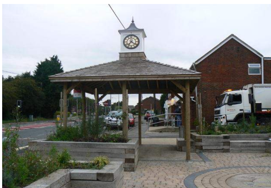
A31 outside the village shops is also identified as danger spot in the survey
